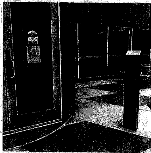
Figure 31: Accessible doors. Door can be automatically opened.
